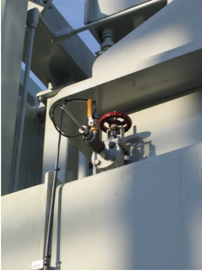
Figure 9: Oil Supply Assy
