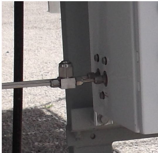
Figure 8: In-Line Oil Filter
