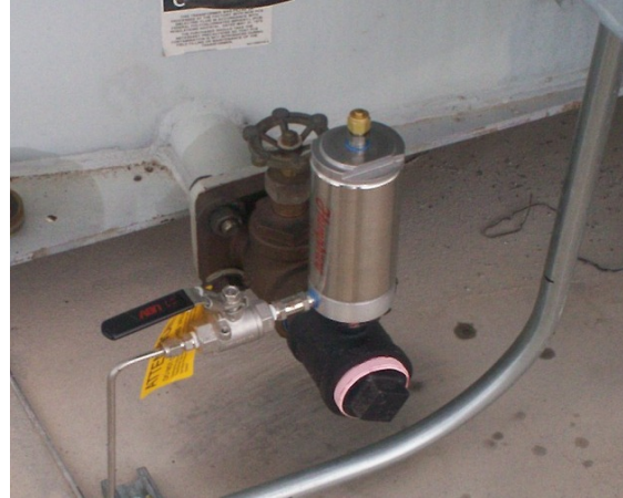
Figure 10: Oil Return Assy / Bleed Fixture
